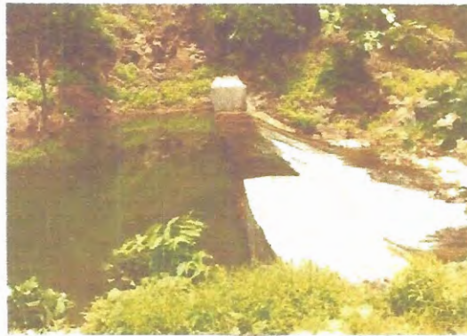
E.13 - Site preparation for B P P at Chopat (1992-93)
