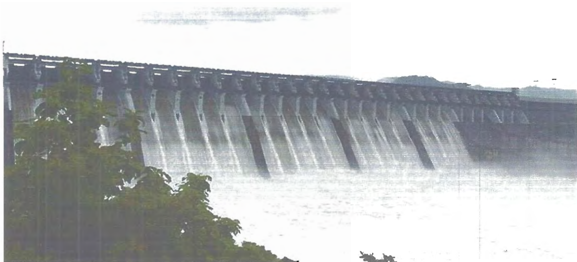
Pic 4. View of Sardar Sarovar Project with open spillway gates
