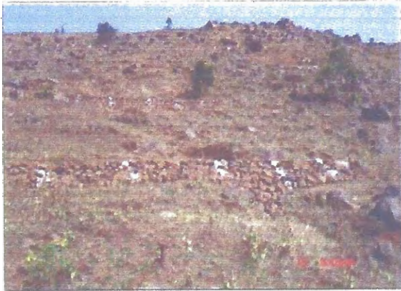
Loose boulder check dam in area of Dhadgaon
