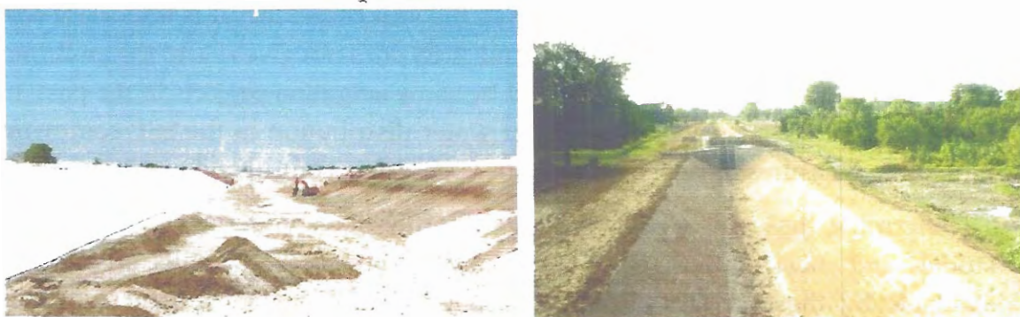
Pic 18. Mechanized lining adopted in canal system of Sardar Sarovar Project
