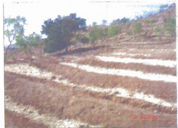
Continuous contour trenches in Dhadgaon
