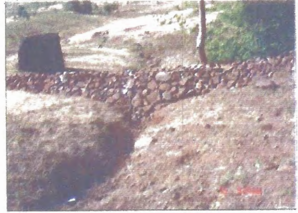
Loose boulder check dam in area of Dhadgaon
